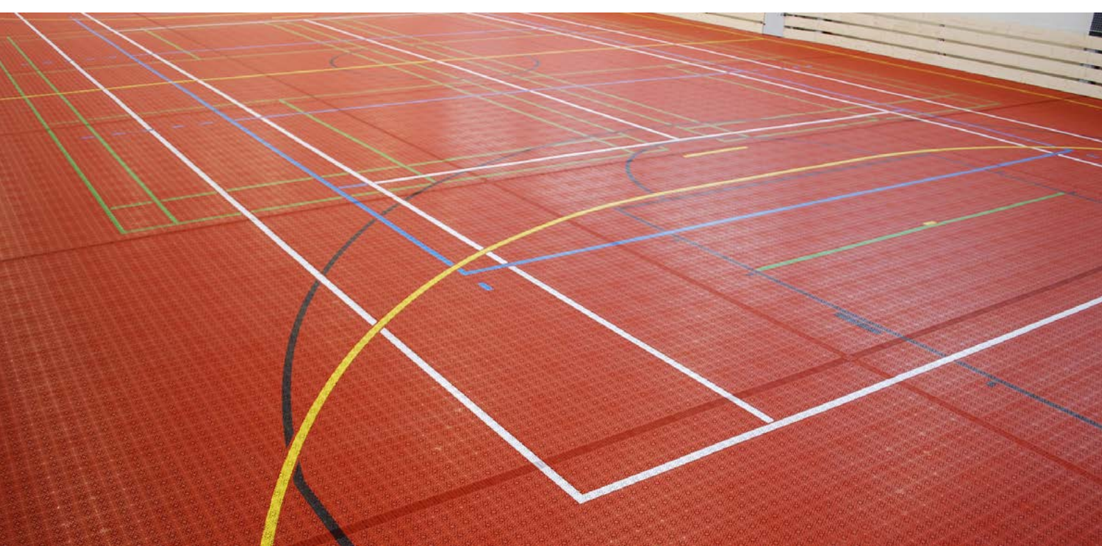
Bergo Tennis gives the right bounce over the whole track. 11° angle of incidence gives a 13° angle of the ball.
